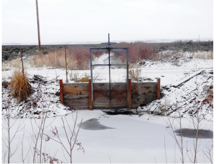
**This outdated manual headgate will be replaced with an automated SCADA controlled headgate paid for in part by a 2016 WaterSMART grant.**
